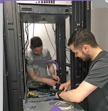
Seriu engineers Tom & James installing Myerson's new server into the rack.
